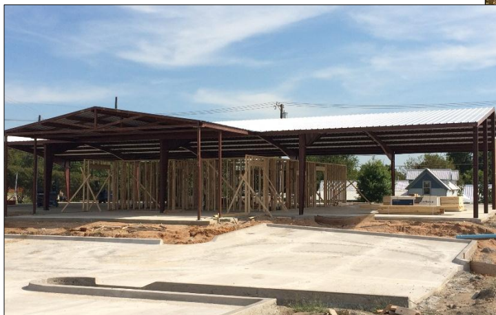
Beginning of framing the inside.
